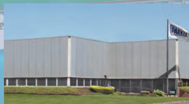
Manufacturing Facilities Fairfield, NJ U.S.A.
